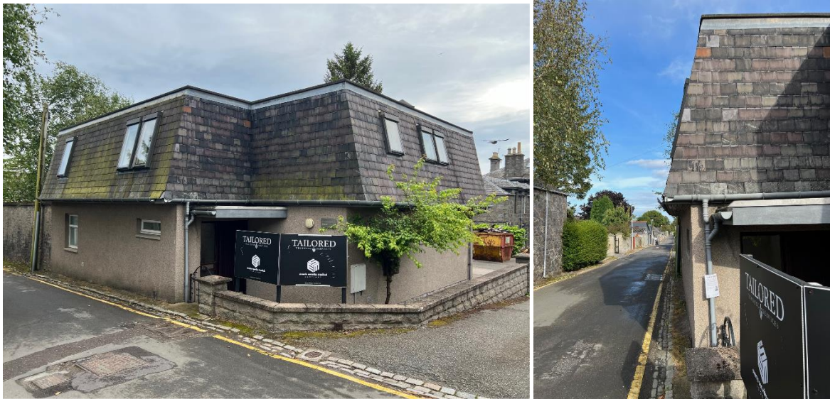
Figure 3 – Existing Office Building
